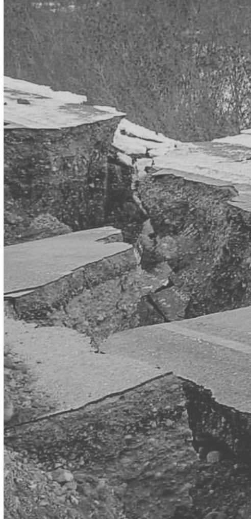
Road damage from the November 3, 2002 Denali Fault earthquake.
