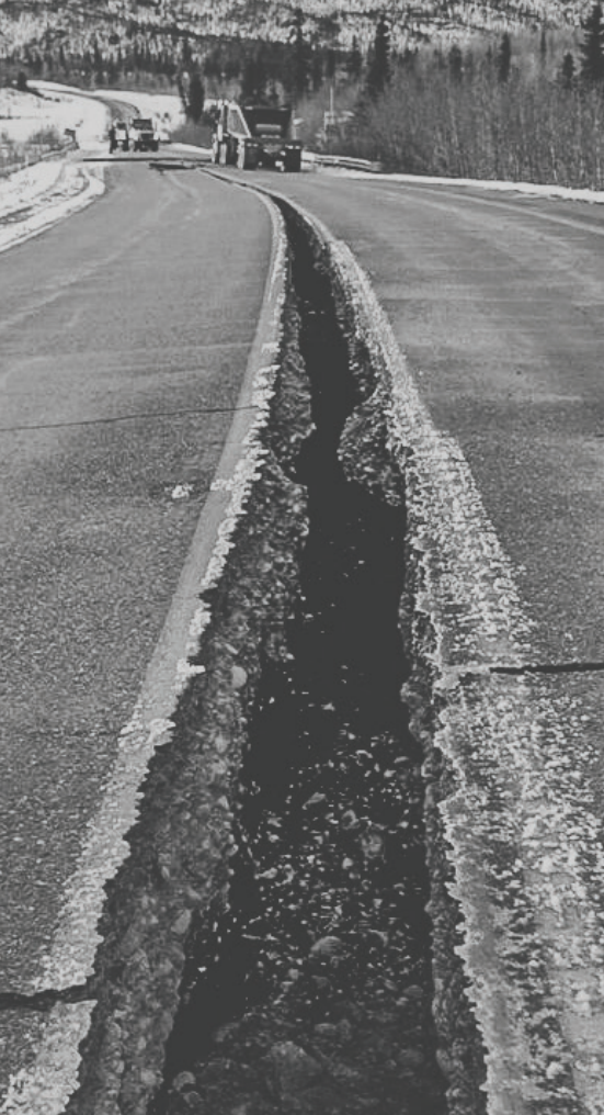
Road damage from the November 3, 2002 Denali Fault earthquake.
